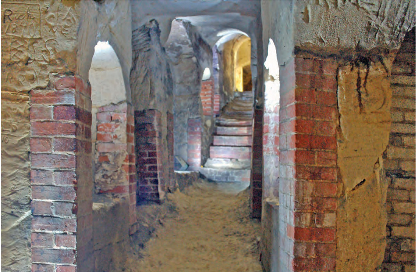
The heavily bayed and alcoved tunnel beneath the Wheatsheaf
